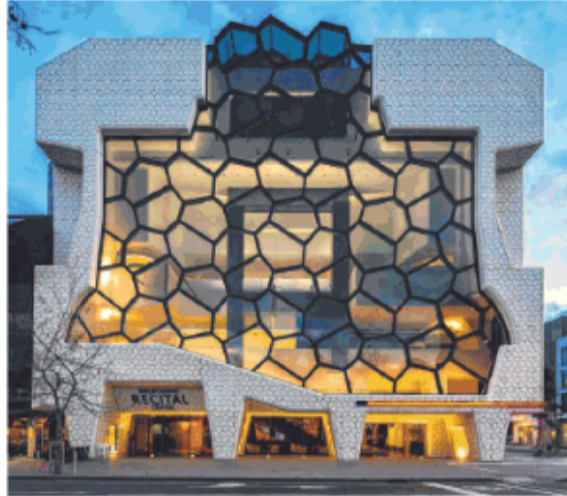
VISIONARY: Architect Ian McDougall led the design team for the Melbourne Recital Centre.
